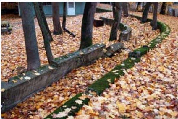
Remains from the Shoot-the-Chutes lagoon structure. This is the point where the passengers would disembark the boats after completing the ride. The boats would splash down into the left edge of this picture.
