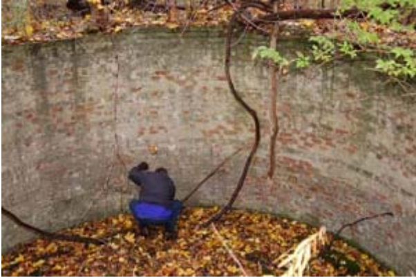
Another view of the cistern.
