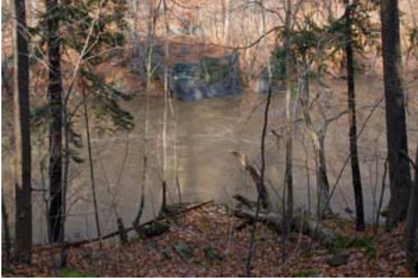
Site of the lower footbridge over the Connoquenessing Creek. Photo is looking toward the north shore (Rock Point side) of the creek.
