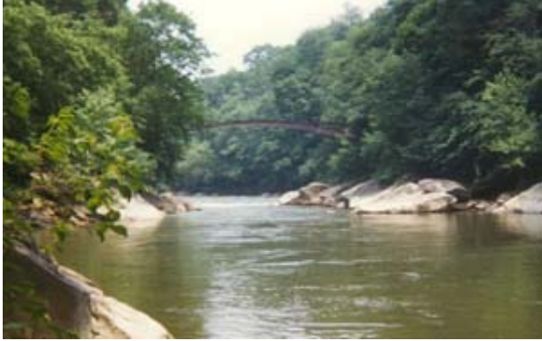
A view of the remnants of the upper bridge taken in 1994. The bridge had no floor decking at this point and was impossible to cross. A large tree fell onto the weakened steel structure, and collapsed it into the creek several years after this picture was taken.
