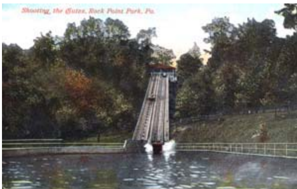
At approximately 300 feet in length , and with a drop of approximately 100 feet (for a down-angle of about 20 degrees), the Chutes, also known as the Toboggan ride, was sure to thrill. [how it looks now]
