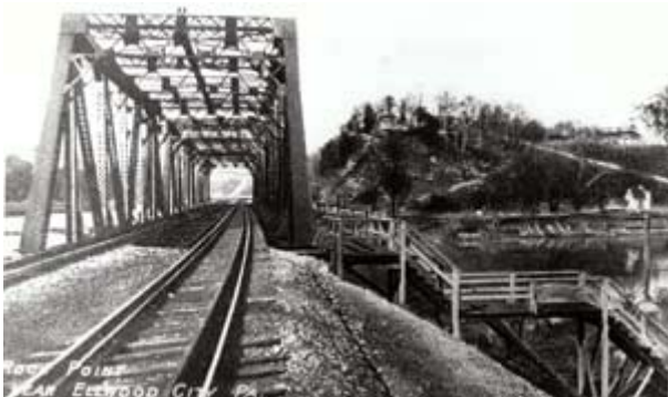
The PY&ARR bridge across the Connoquenessing Creek - the park can be seen in the background. This scene was taken looking north, with the Beaver River on the left, and the Connoquenessing Creek on the right. Note the walkway area of the bridge which would enable pedestrians to cross the creek to the park.
