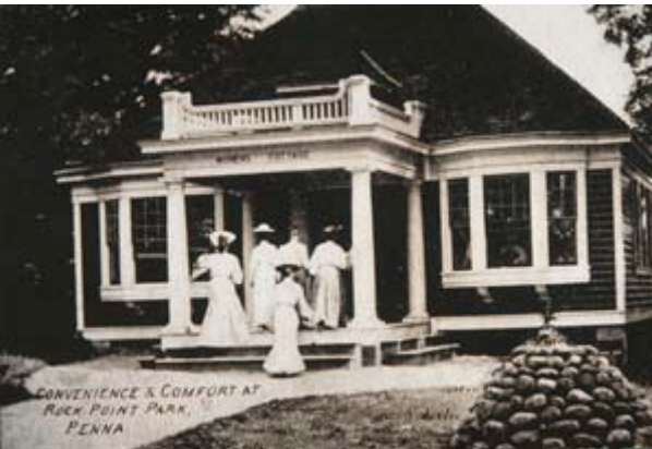
The "Womens Cottage" - a luxury refreshing station for women, it was the main Ladies restroom for the park. It was situated on the bluff, near the top of the Shoot-the-Chutes ride. [how it looks now]
